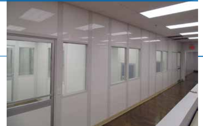
Cleanroom with PVC Wall Finish
