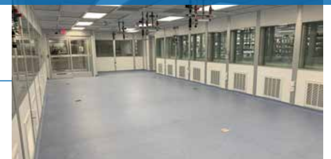
Low Sidewall Return Air Chase Design
