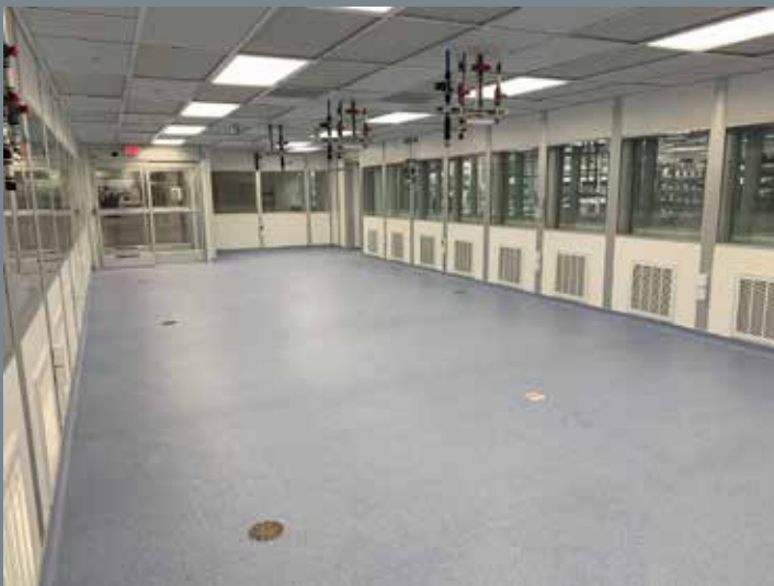
Low Sidewall Return Air Chase Design
