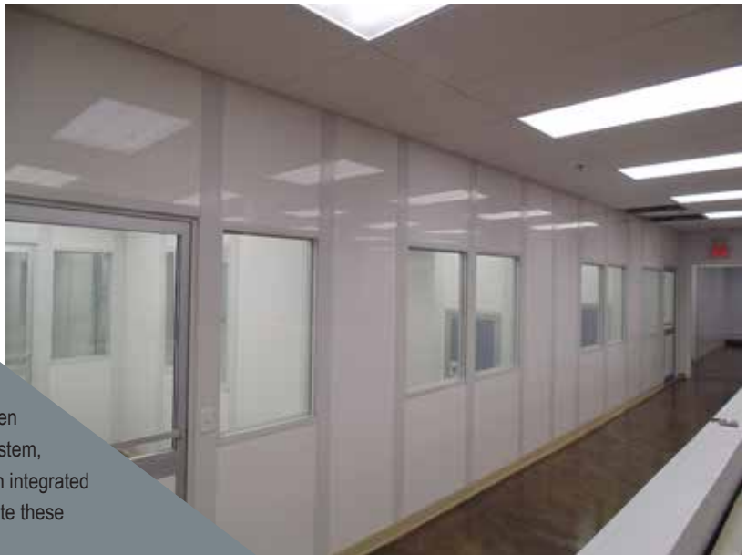
Cleanroom with PVC Wall Finish
