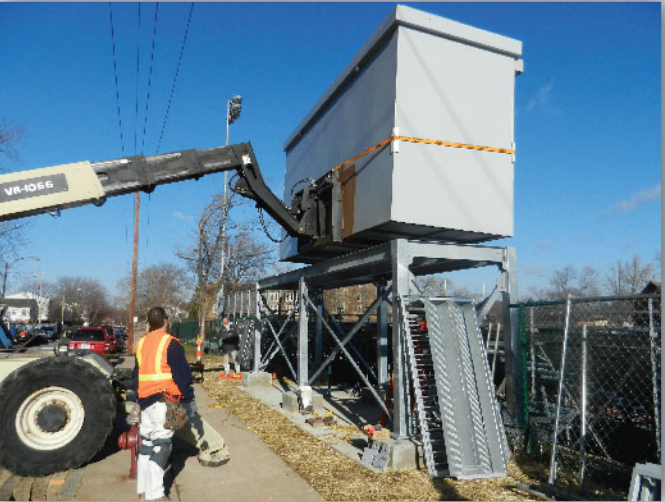
This press box was lifted from the back of the delivery truck and then quickly installed on top of our mezzanine support structure. The entire installation, including the platform, was completed in less than two days.
