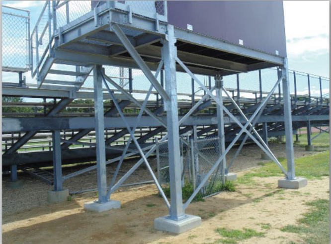
We supplied this galvanized steel platform to create independent support and elevate the press box above the existing bleachers.
