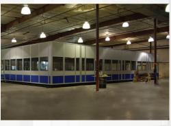
Giant structures like this 30' x 60' office complex are shipped to site in smaller factory assembled modules where they are easily joined together to create the finished structure.
