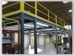
Mezzanines: Storage Platforms, Equipment Platforms, Conveyor Crossovers and Fall Protection Platforms. Heavy-duty structural steel components designed in accordance to IBC building code.
