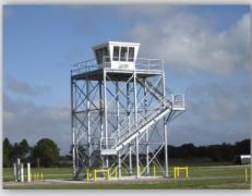
Prefabricated Towers: Guard Towers, Range Towers, Observation Platforms and Rappelling Platforms. Corrosion resistant galvanized steel construction provides years of trouble free service for these and other custom tower applications.
